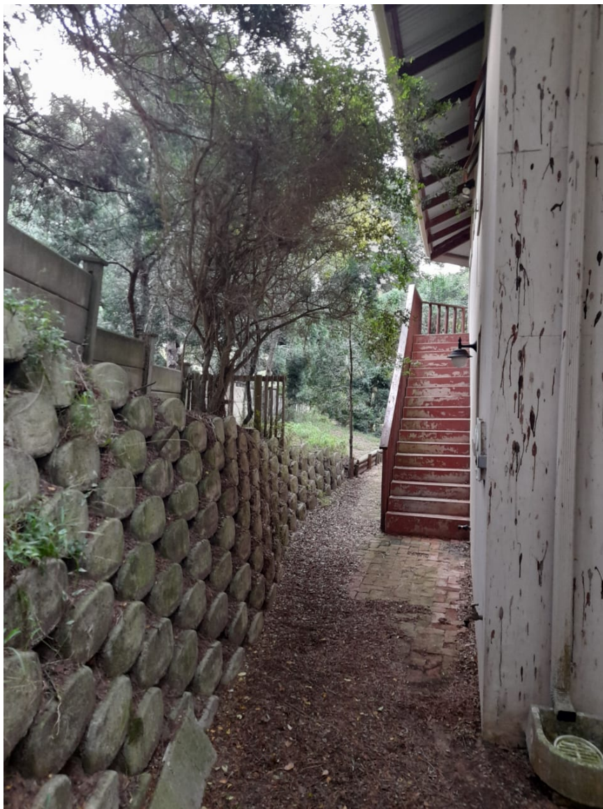
Figure 4: View of existing concrete block retaining wall
