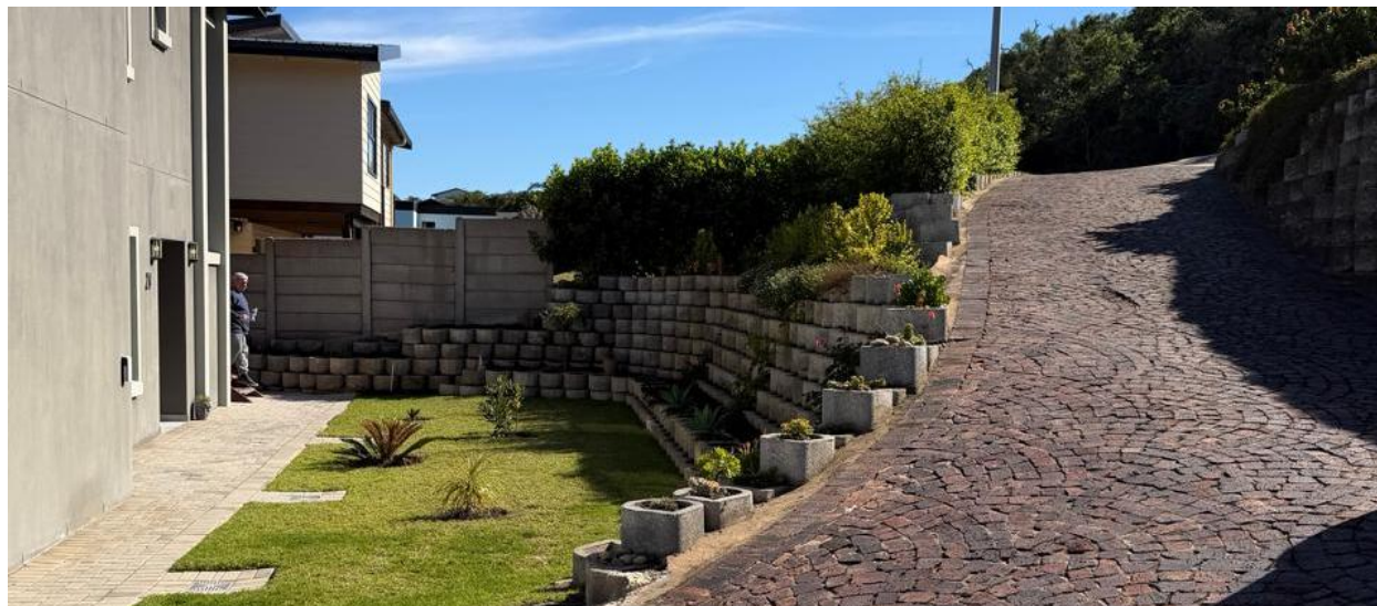
Figure 4: Image of as-built retaining structures
