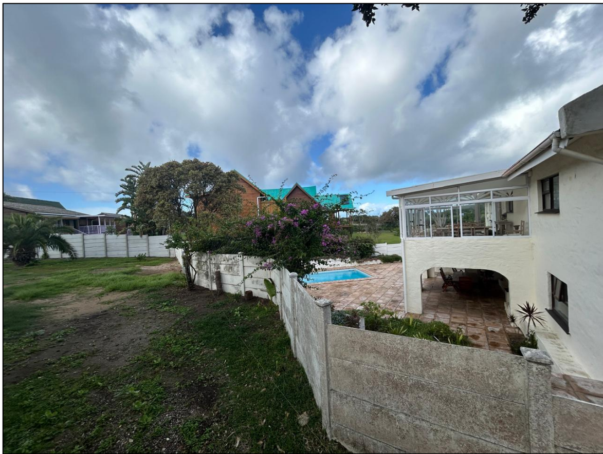
FIGURE 1: STRUCTURES ENCROACHING BRENTON ERF 254
