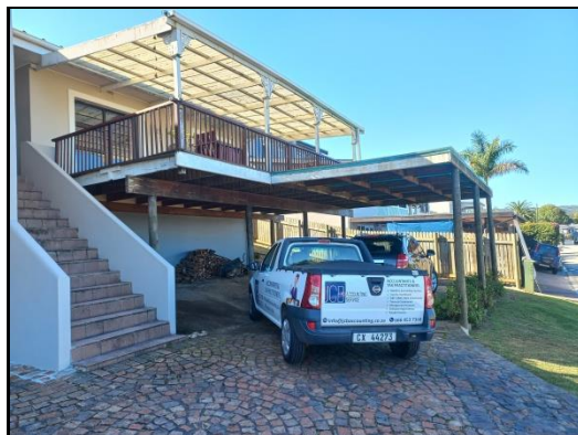
Fig 2: As-built carport and roof section over street building line.
