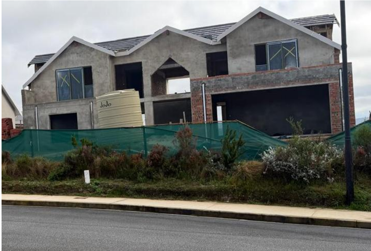
Figure 5: Subject dwelling with complete roof on 17 June 2026
