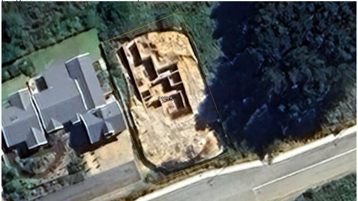
Figure 4: Walls almost complete on 3 November 2025 (photo courtesy of Google Earth)
