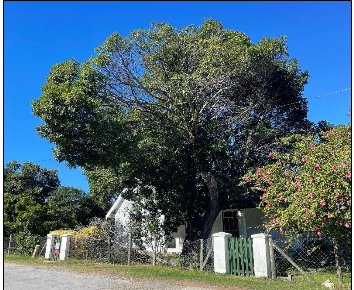
Figure 2: Existing Milkwood Tree.
