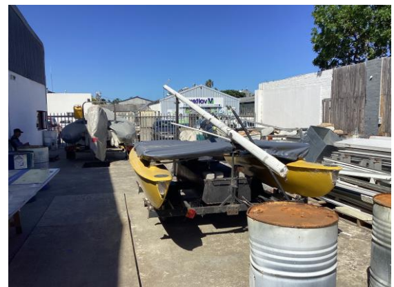
Plate 7: Proposed construction area, Phase 1A, within Erf 3417, within courtyard area, looking towards entrance road. This area will be roofed.
