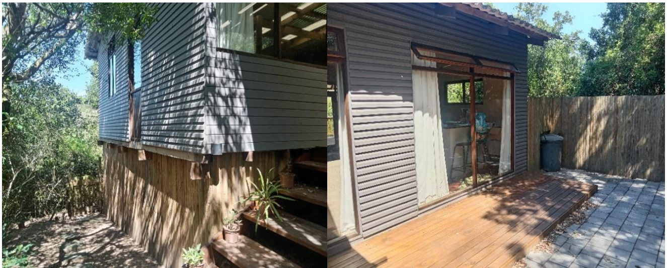
Figure 4: Existing Additional Dwelling Unit.
