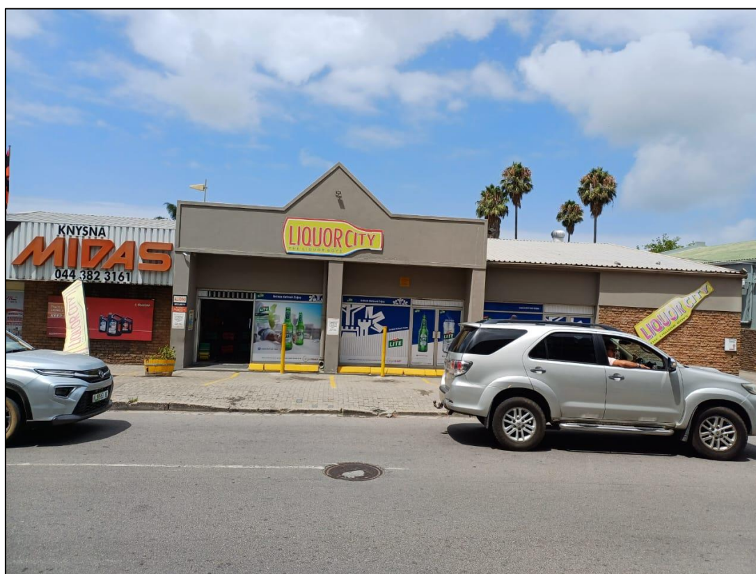
FIGURE 2: EXISTING STRUCTURES ON THE APPLICATION AREA
