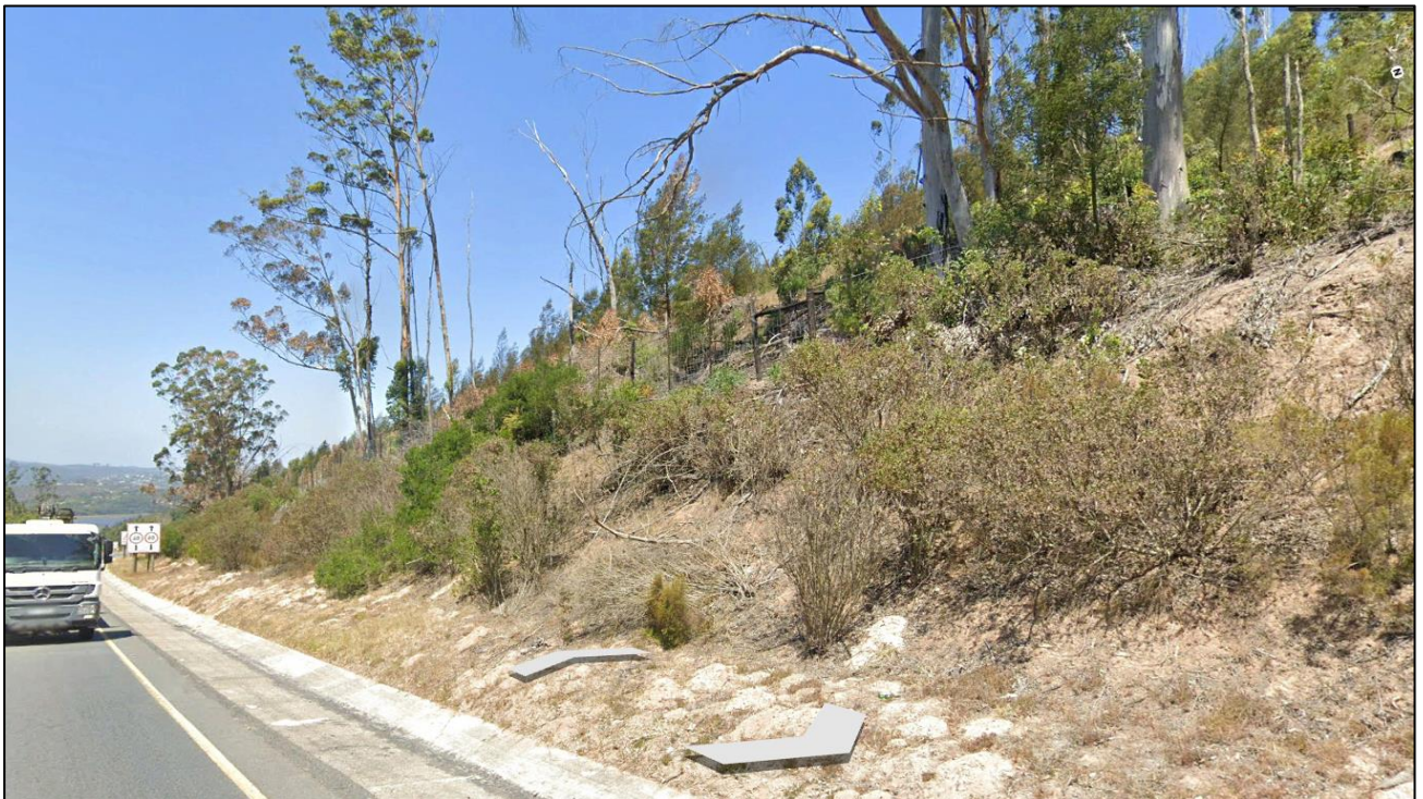
Figure 14: view from the N2 - eastern direction.
