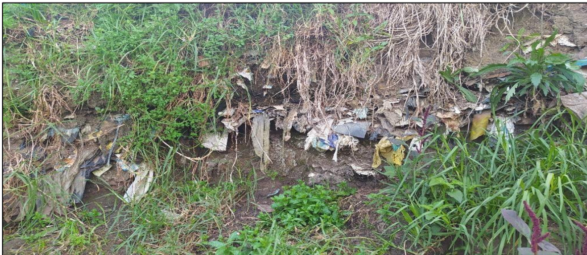
Condition of the imported material
