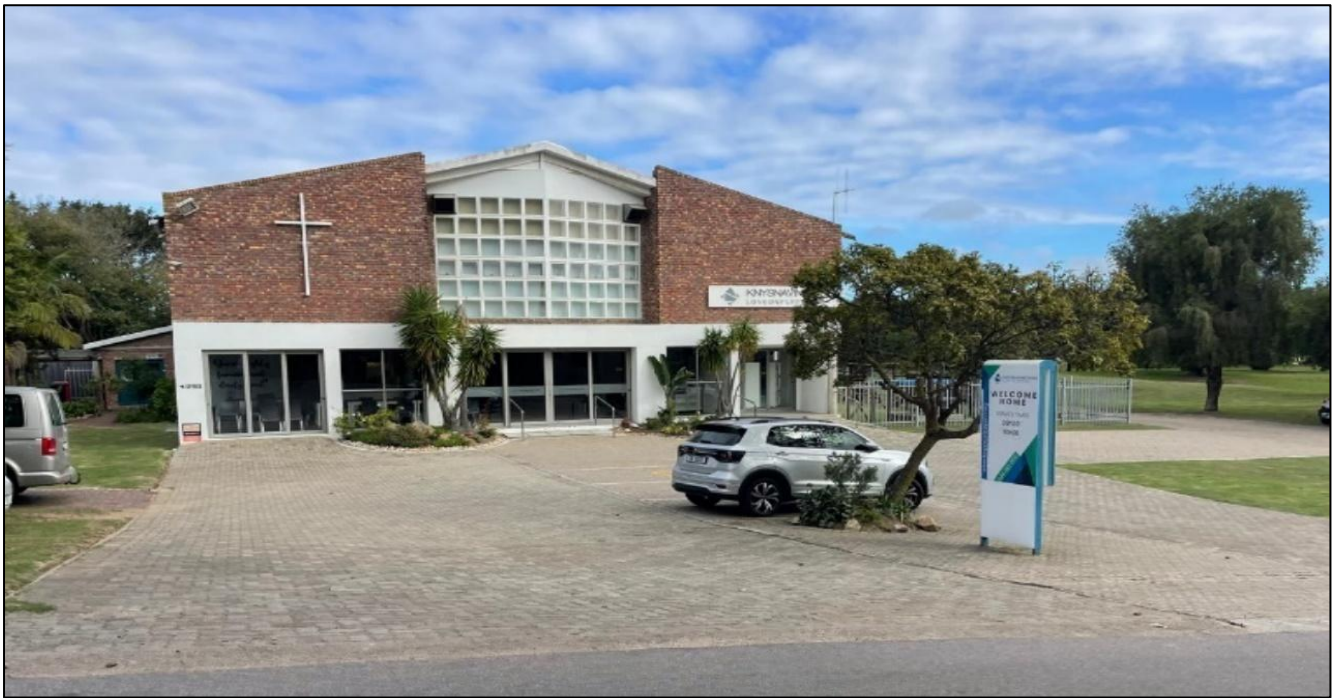
Figure 4: Existing Church Building.
