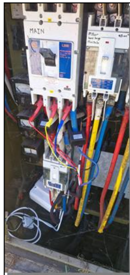
Fig.6) Picture of DVM' Landis & Gyr Logger clipped onto main 450A MCCB
