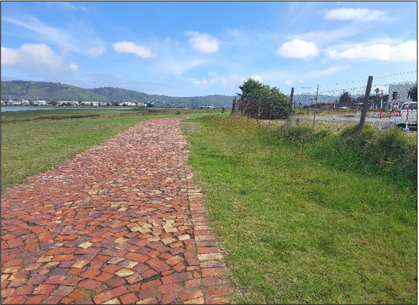
Figure 9: Existing fence around the testing ground (southern boundary).
