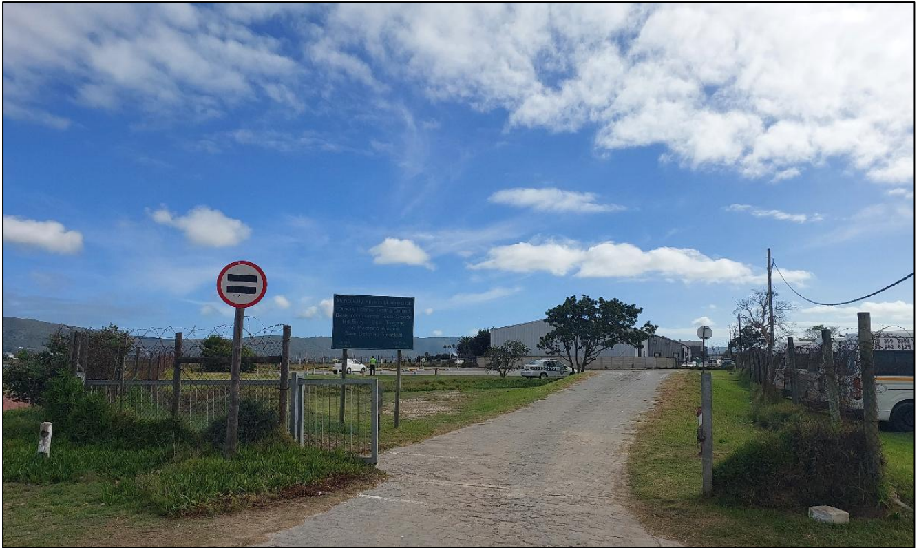
Figure 3: Existing Driver's Licence Testing Facility.
