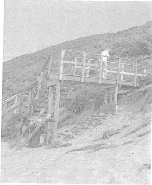
Base of temporary boardwalk showing additional support structures for stability.
