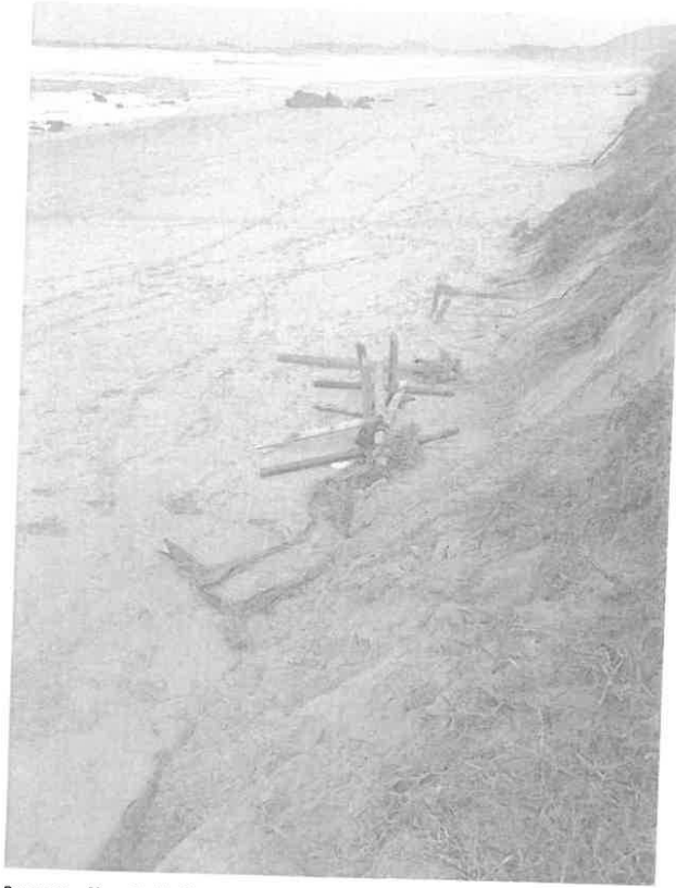
Remnants of boardwalk after storm, steep exposed sandy cliffs prevented safe access to the beach.
