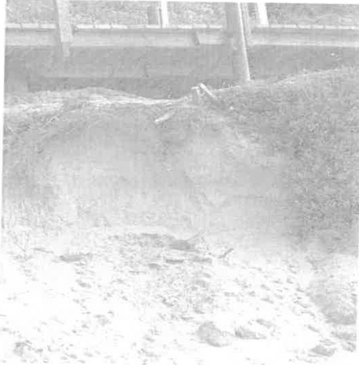
Unstable dune directly beneath the temporary boardwalk
