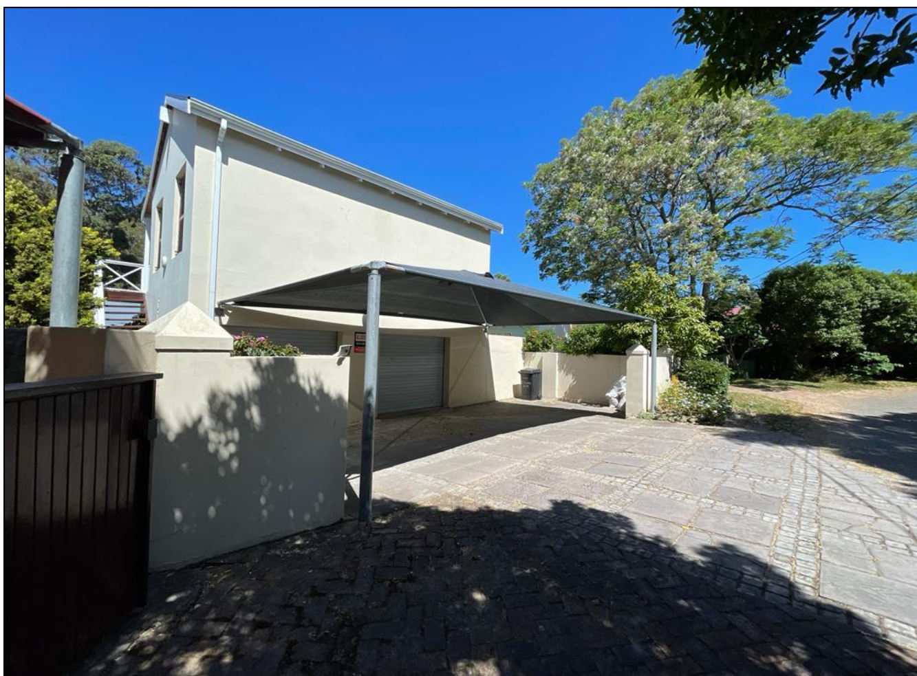
Figure 3: Picture indicating the existing garage, encroaching carport, access.
