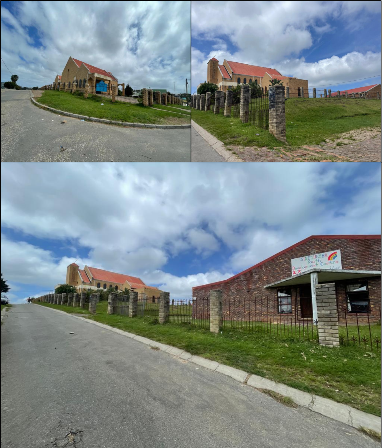
Figure 3, 4 & 5: Pictures indicating vegetation, slope and structures on site.
