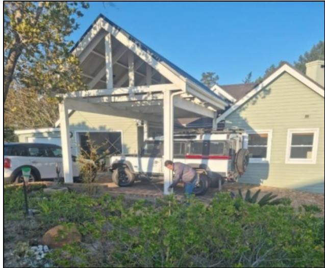
Figure 6: Encroaching Porte Cochere.
